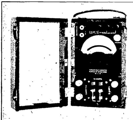
FIG. 108.—Volt-ammeter employing the current transformer
